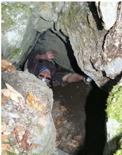
Bruce in collapsed adit
